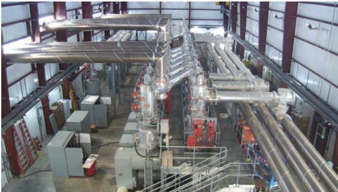
Gas Insulated Switchgear mounted indoors
