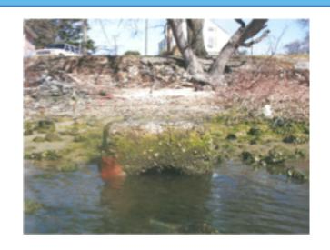
Undersized, outdated stormwater pipes were installed so long ago they are underwater at *low* tide! Stormwater solutions must involve holding water and infiltrating.
