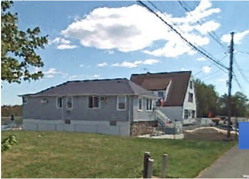
Current Building Practice
