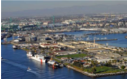
$700,000 replacing pier facilities
