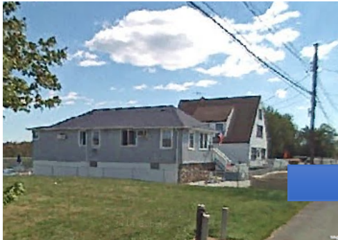
Current Building Practice
