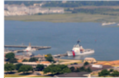
$1.7M to replace HVAC
