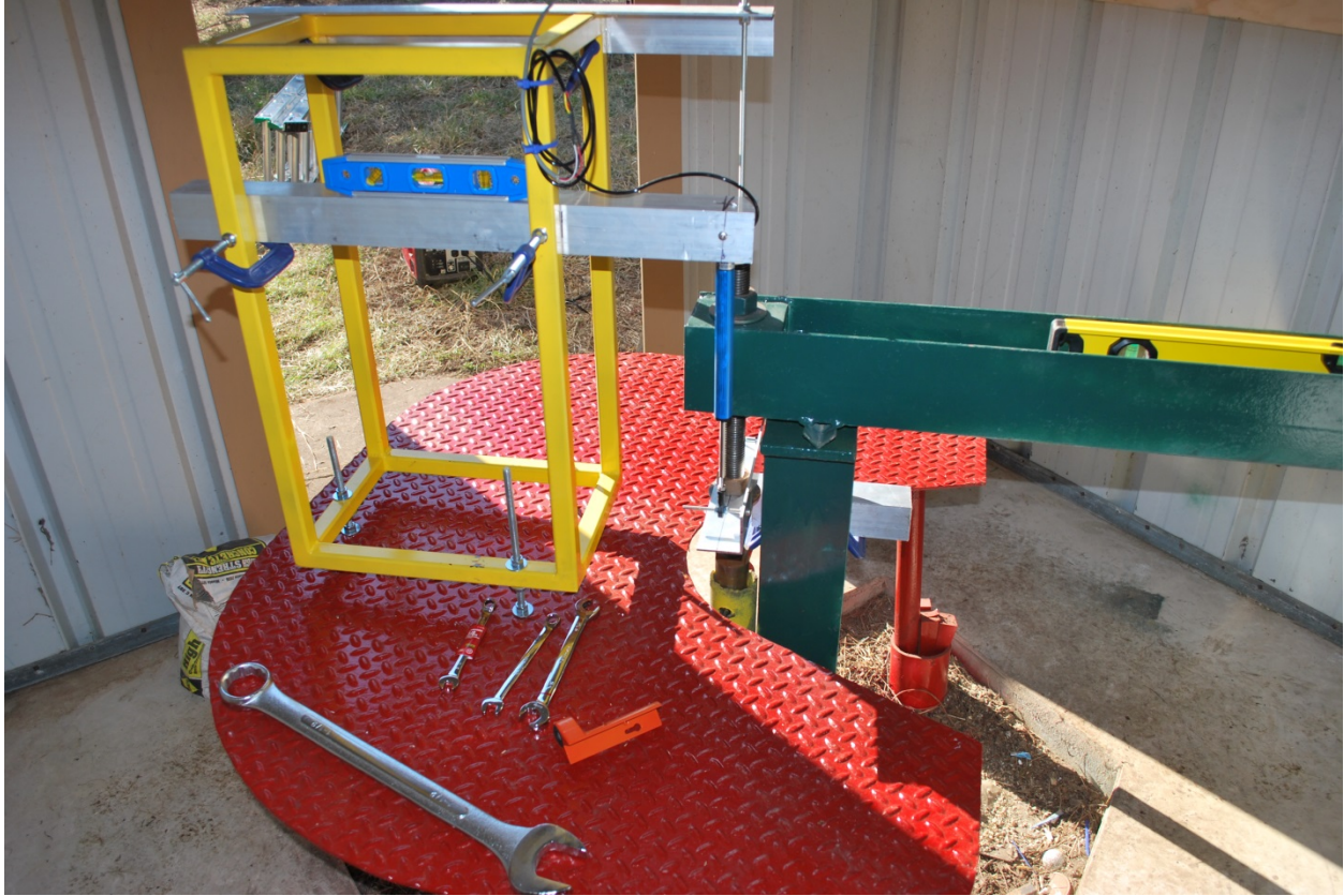
Figure 3. Installation of new equipment and a digital potentiometer on the Suffolk extensometer (58C 52). Photograph by David Nelms, February 18, 2016.
